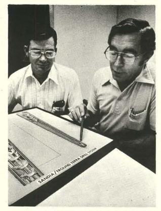
TERRA DRILL SYSTEM concept is reviewed by inventors Bob Alvis (5715) and Max Newsom (5735). The rotary bit is fitted to fire bullet-like projectiles to break up hard rock strata.
